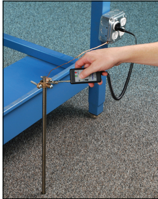
Figure 5. Testing auxiliary ground with the 19249 tester
