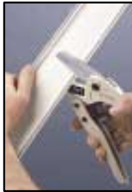
Cut cover to desired size.
