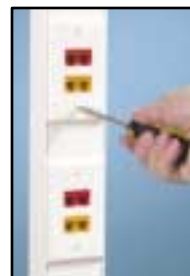
Install faceplate over bracket.
