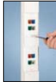
Install faceplate over module frame.
