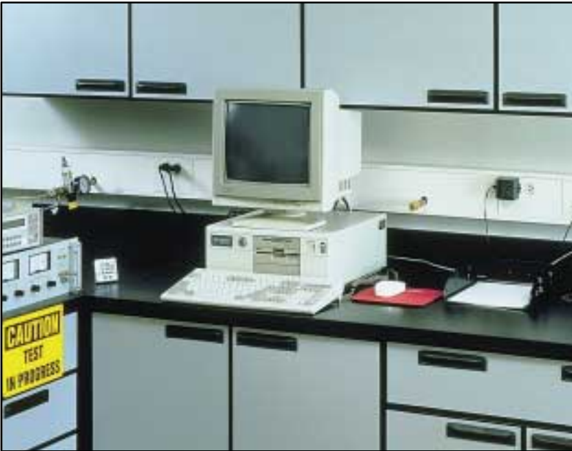
With a large capacity and multichannel capability, PAN-WAY Type T Surface Raceway can integrate both power and communication cabling systems while maintaining a neat and professional appearance throughout a testing lab.
