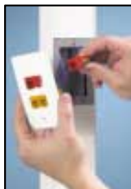
Terminate jacks and snap jacks into faceplate.
