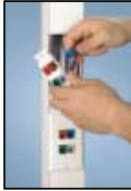
Terminate jacks and snap into module frame.
