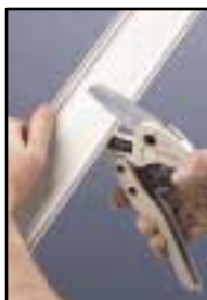
Cut cover to desired size.
