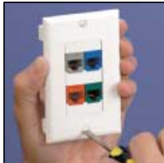
Screw module frame and faceplate together...
